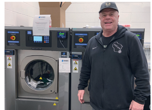
Herd Equipment Manager Mike Sergo stands in front of the Menominee Nation Arena's new Sports Laundry System washer-extractors. They work seamlessly with ozone injection to disinfect athletic laundry.
