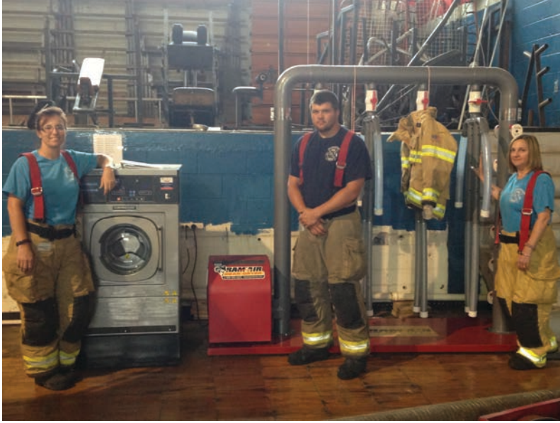
Firefighters at Cordova Fire Dept., in Cordova, Ala., stand next to their Continental ExpressWash Washer-Extractor and ExpressDry Gear Dryer. The equipment was installed on an old high school basketball court after two tornadoes destroyed their fire station.
